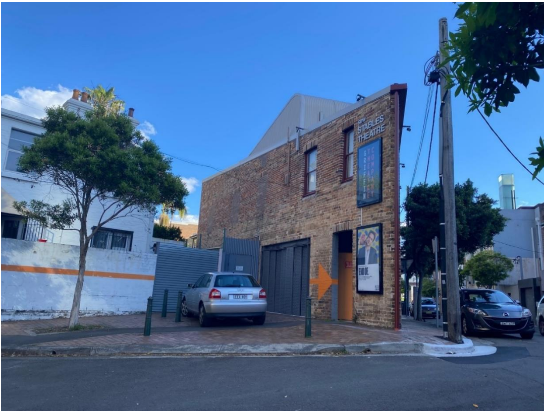
Figure 3. 10 Nimrod Street, viewed from the north-west
